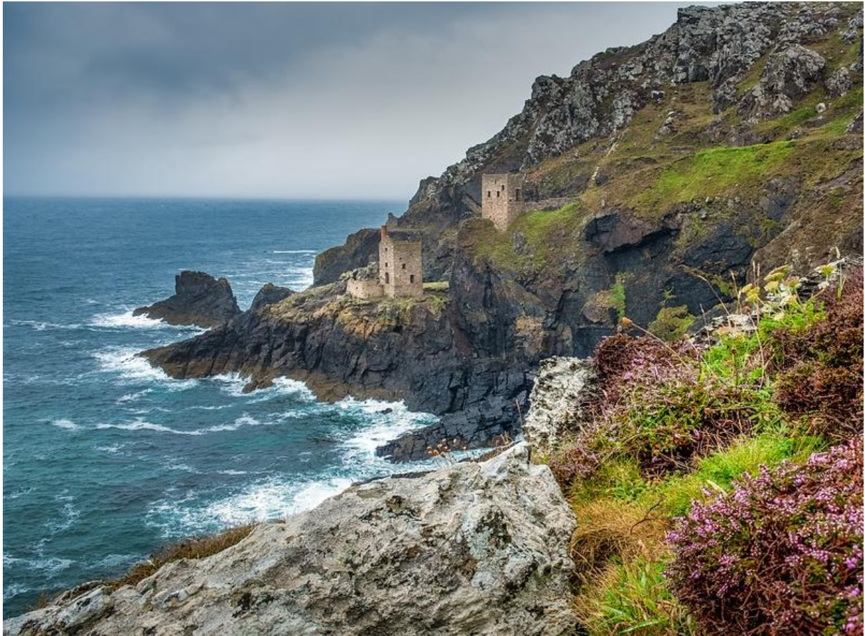
Reference Image: Crown Engine Houses at Bottalack, Cornwall
